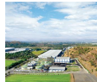
Jain Energy Park Jalgaon (Maharashtra) Solar & BioGas
