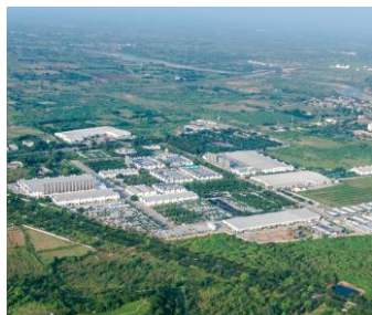
Jain Plastic Park Jalgaon (Maharashtra) Micro Irrigation, Plastic Piping & Sheet
