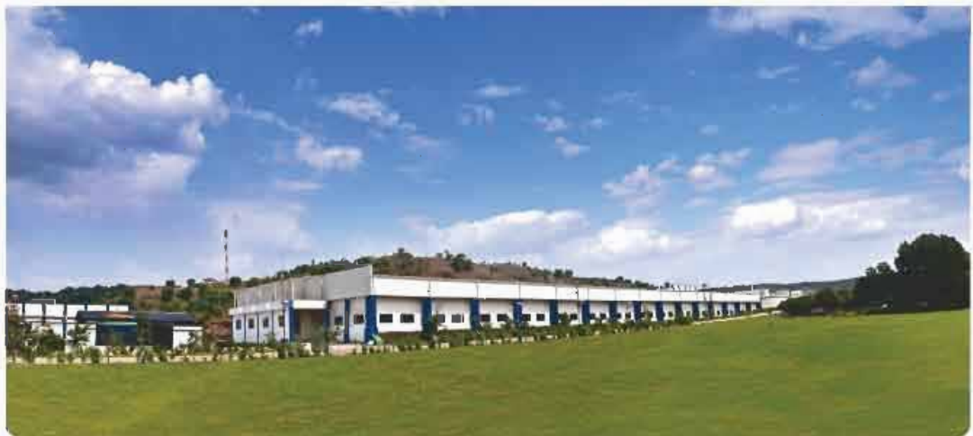
Solar Products : Jain Energy Park, Jain Valley, Jalgaon, Maharashtra (India)
