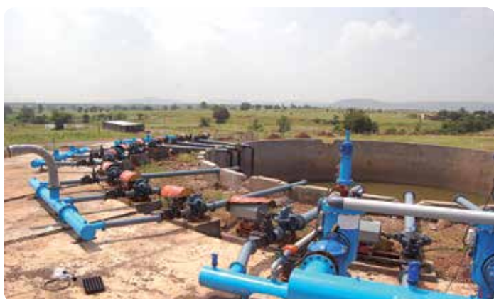
Jain fully automatic Filter station. Subsurface Drip Irrigation Project at Sampatrao Deshmukh Sahakari Pani Puravtha Sanstha Raigaon, Sangli. In this project, water is proposed to be lifted from Hingangaon Talav which is fed by Tembhu Lift Irrigation scheme. Water from Hingangaon talav is lifted by 4.16km 900mm HDPE rising main and delivered into Main Delivery Chamber of 2000cum capacity. Secondary pumping and Centralised Self-cleaning filtration unit is proposed at MDC. From secondary pumping unit primary HDPE/PVC pipe distribution network is proposed to the block level. (Block of approx. 40-45 acre area). From Block level secondary PVC piping network is provided up to the farm level. Sectional (each section is of approx. 4 acre area) automated drip system is provided at farm level and total area of 2009 acre is covered under subsurface drip irrigation.
