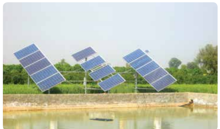
3HP DC Solar submersible pumps for irrigation purposes installed for marginal farmers in Rajasthan.
