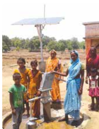
Solar hand pumps installed in rural and backward areas of Madhya Pradesh for drinking water purposes.
