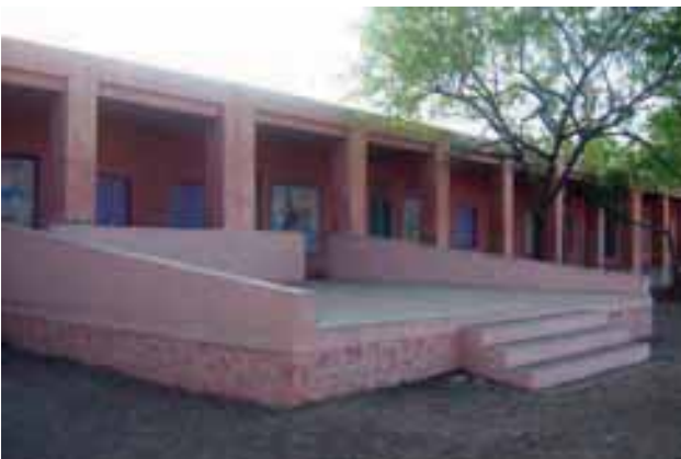
Lending a helping hand; the renovated building of the Zilla Parishad Urdu School, Shirsoi
