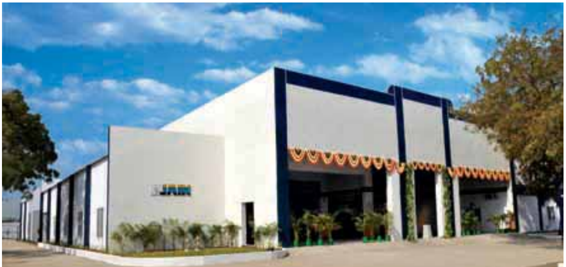
Micro Irrigation Systems and Plastic Piping : Jain Plastic Park, Bhavnagar, Gujarat (India)
